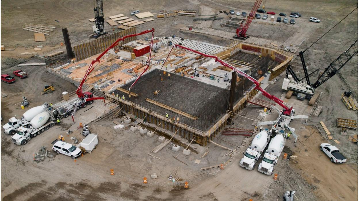
*June 9, 2023: Red River Structure: Final of 4 mass concrete placements for 10-ft thick structure slab; also the largest concrete placement for the entire FMM Project. Photo from C Three Media*
