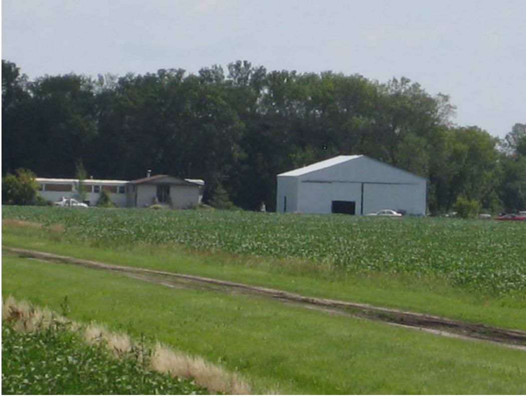
Figure 9 – Parcel No. 70000013646010 – junk vehicles, storage buildings. No access granted.
