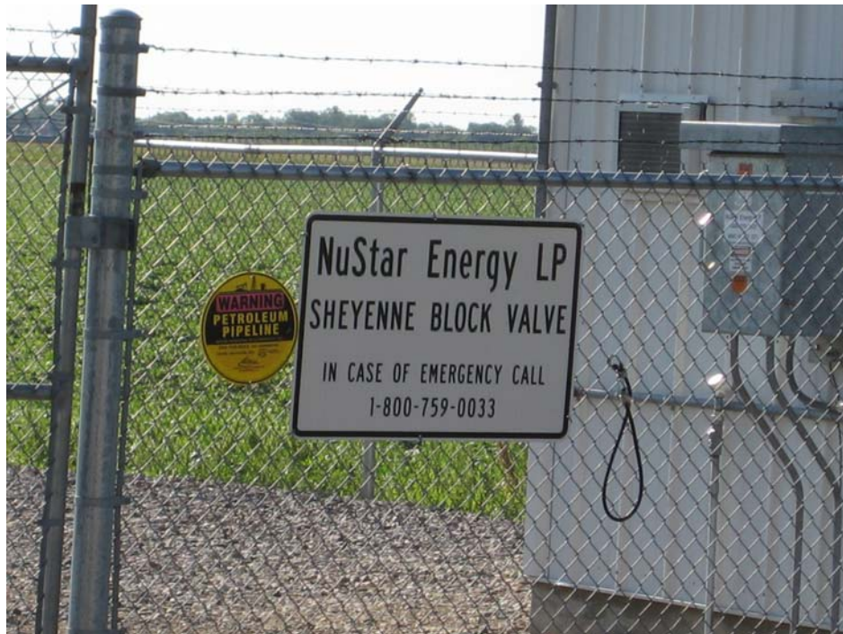
Figure 3 – Substation near intersection of 15 th and 21 st .
