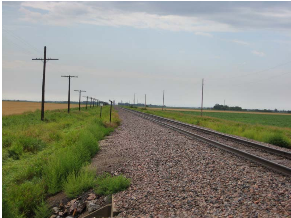
Figure 8 – Railroad tracks near parcel No. 150103000 in Clay County, MN.
