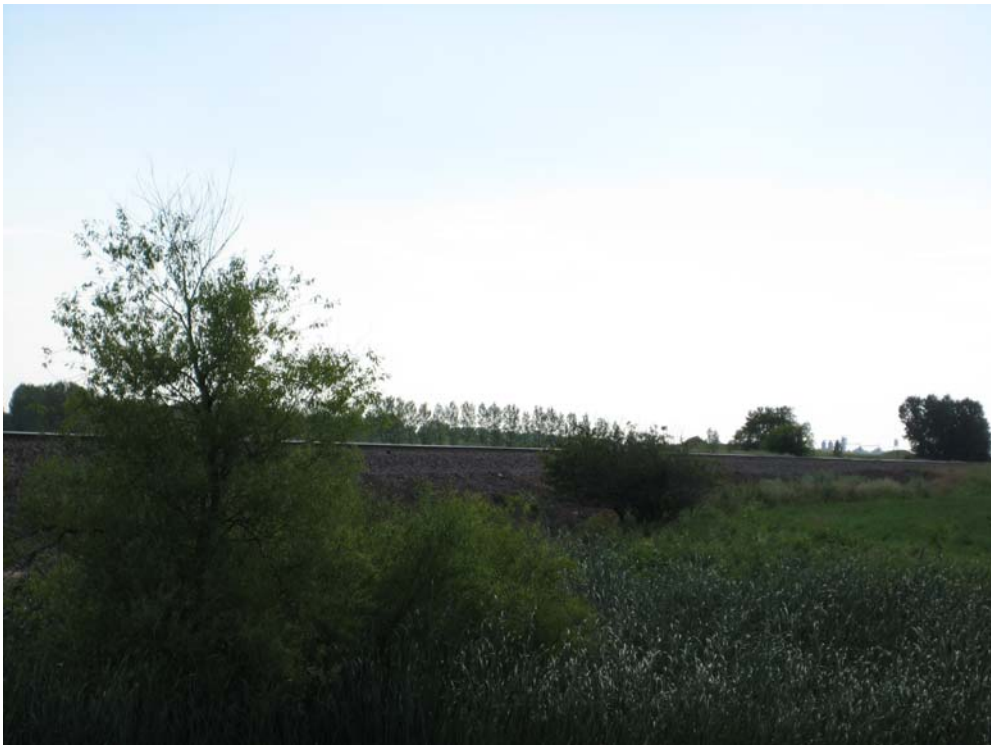
Figure 6 – Railroad at 38 th Street West, north of Interstate 94.
