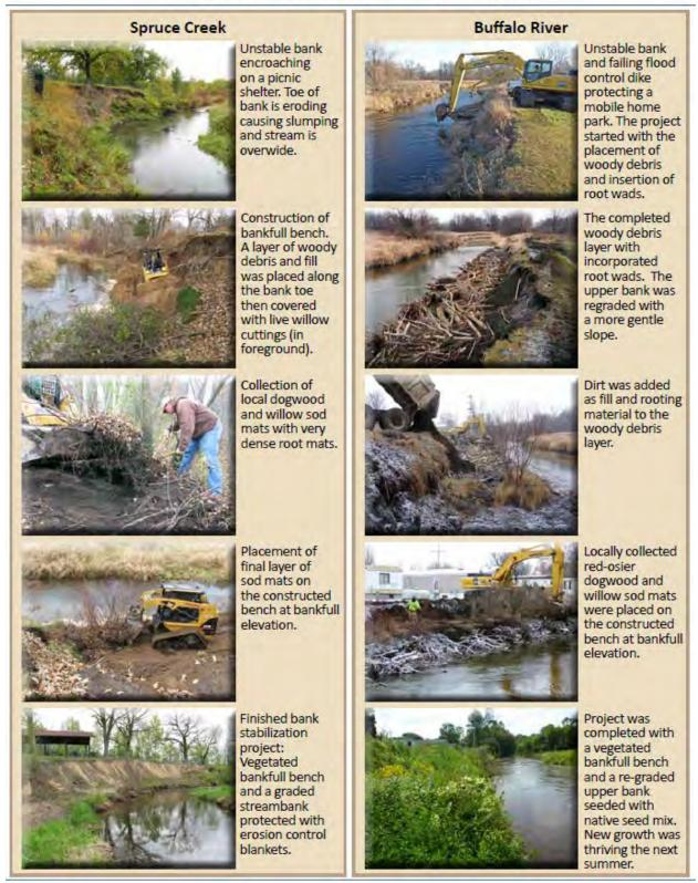
Figure 6-5: Toe Wood-Sod Mat Construction Examples (source: Minnesota DNR)
