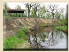
Finished bank stabilization project: Vegetated bankfull bench and a graded streambank protected with erosion control blankets.
