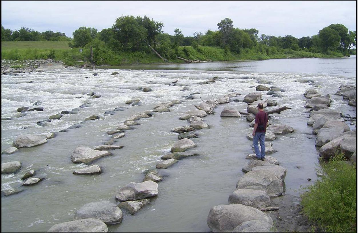
Figure 4. Example of a rock rapids fish passage project at Riverside Dam, Grand Forks, ND on the Red River of the North.
