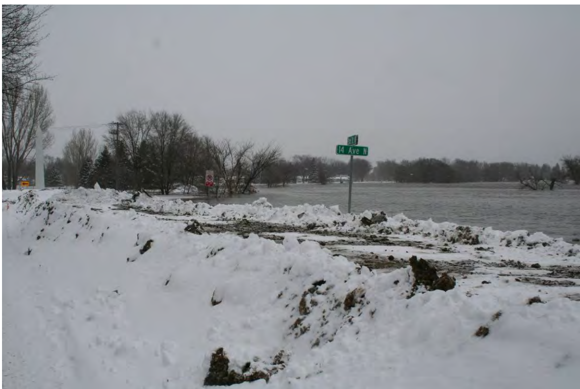
Figure B19. Temporary dike along RRN at Elm St. and 14th Ave. N. in Fargo on 3/26/2009. . RRN stage at Fargo): 39.6 ft (Photo Courtesy of North Dakota State University)
