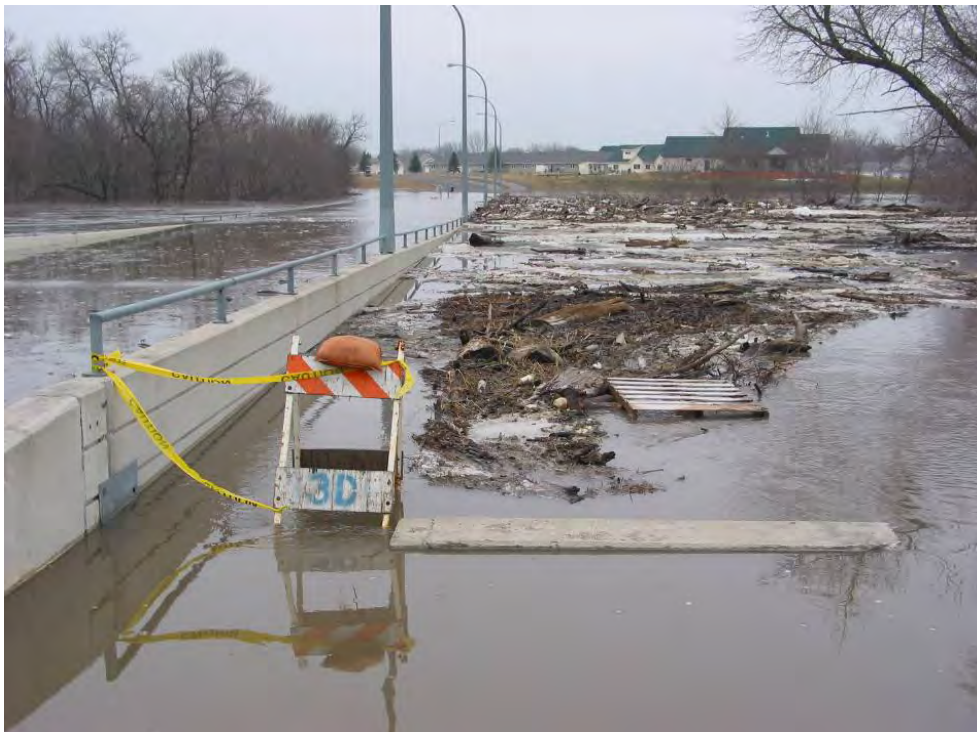
Figure B10. Debris jam at flooded 12th Avenue N. Bridge in Fargo on 4/2/2006. Red River stage at Fargo was 31.9 ft. (Photo Courtesy of North Dakota State University)
