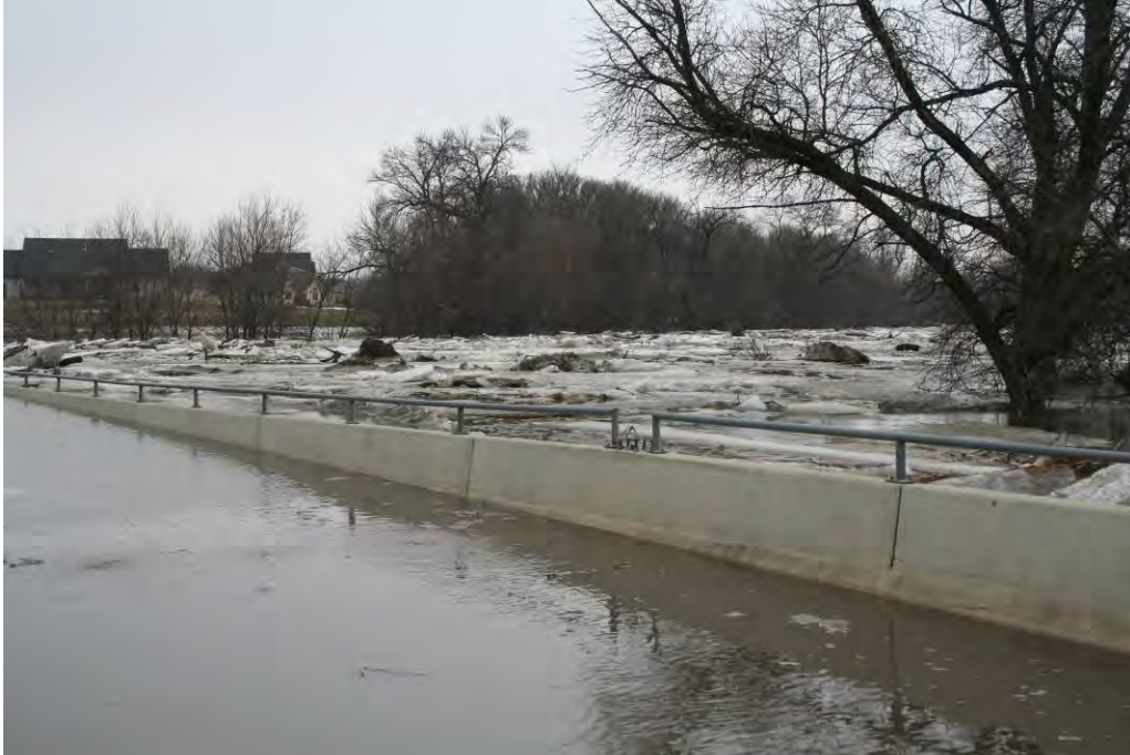
Figure B16. Ice and debris jam at 12th Avenue N. Bridge in Fargo on 3/24/2009, RRN stage at Fargo: 32.4 ft. (Photo Courtesy of North Dakota State University).
