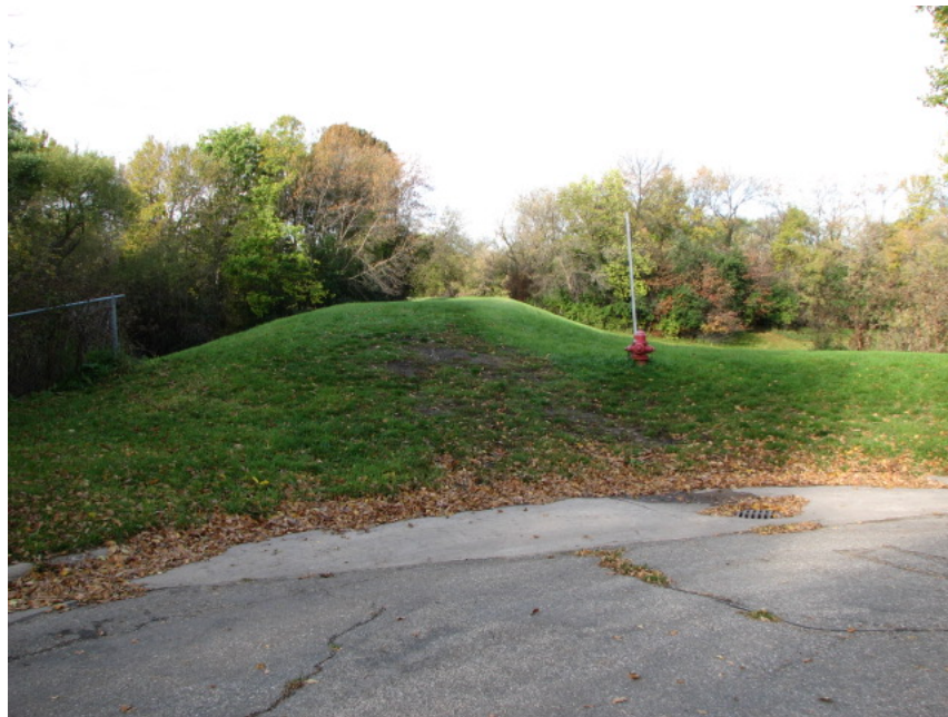
Photo 14: North end of levee. An emergency levee is required to be constructed to tie existing levee into high ground.
