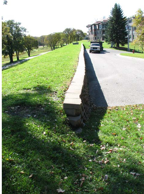
Photo 5: Retaining wall constructed in dryside of levee. Residential buildings located adjacent to dryside of levee.
