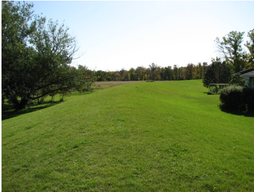
Southwood Drive Levee
