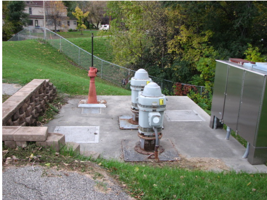
Photo 11: Pumpstation located within levee.
