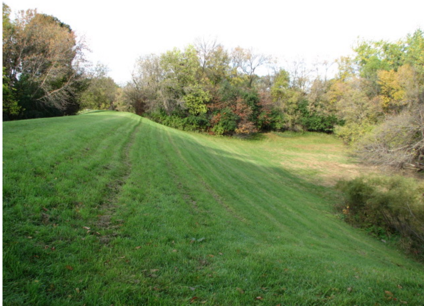
Horn Park Levee
