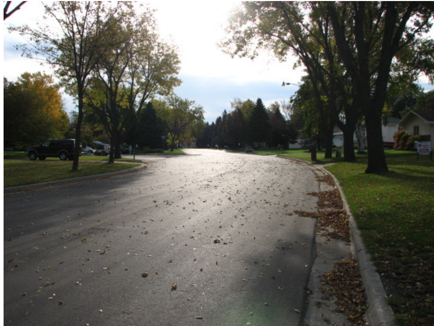
Horn Park Levee
