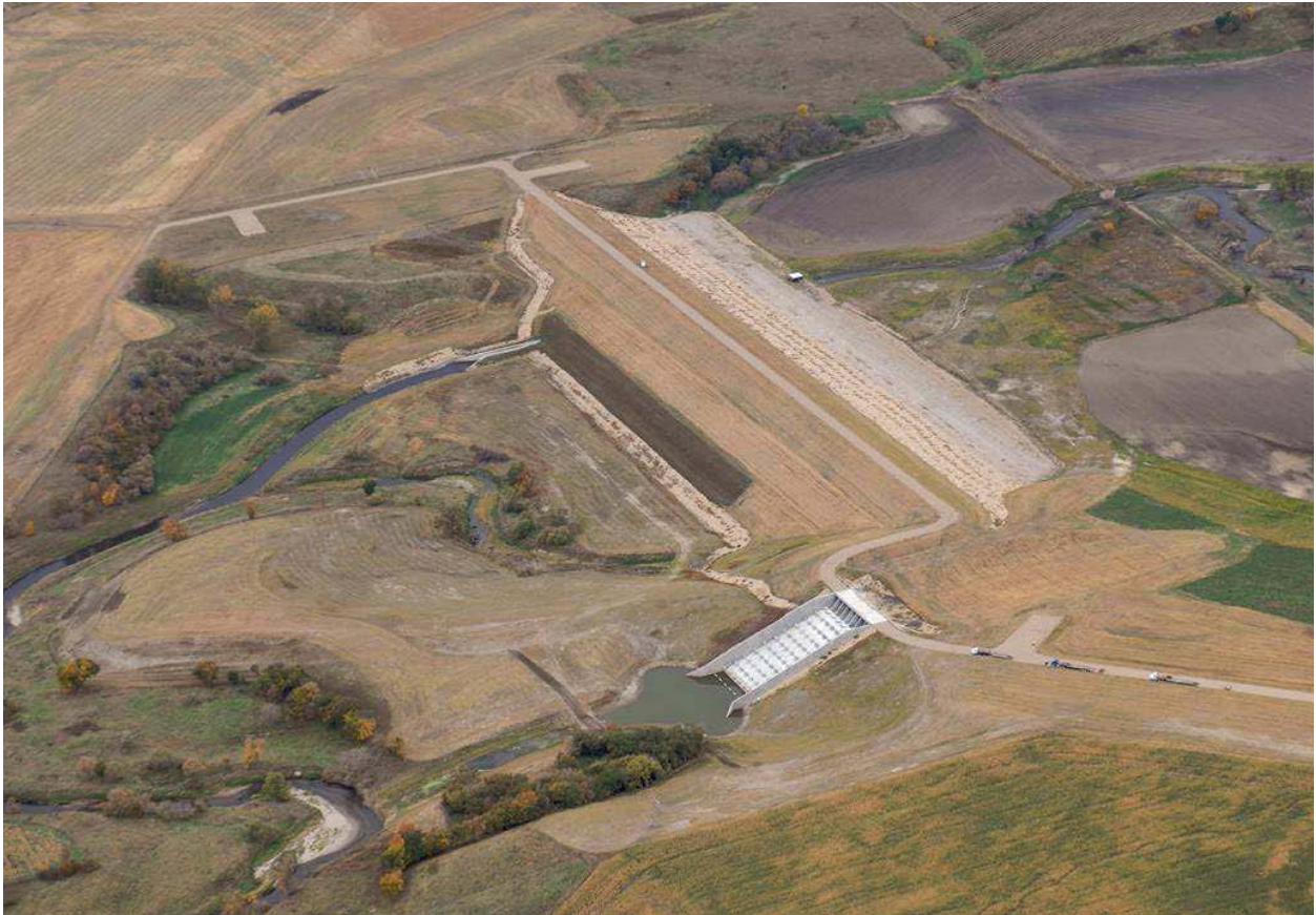
Figure 8. Maple River Dam (Source: Moore Engineering)
