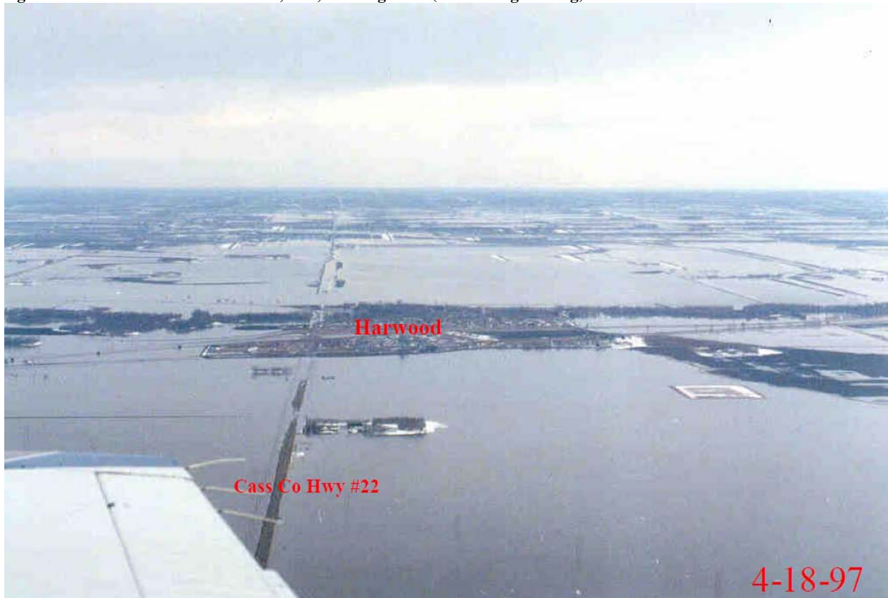
Figure 19. Breakout flows at Harwood, ND , Looking West (Moore Engineering)
