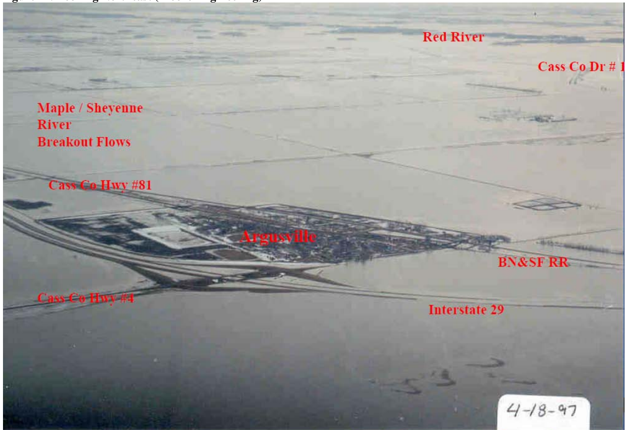
Figure 22. Looking Northeast (Moore Engineering)
