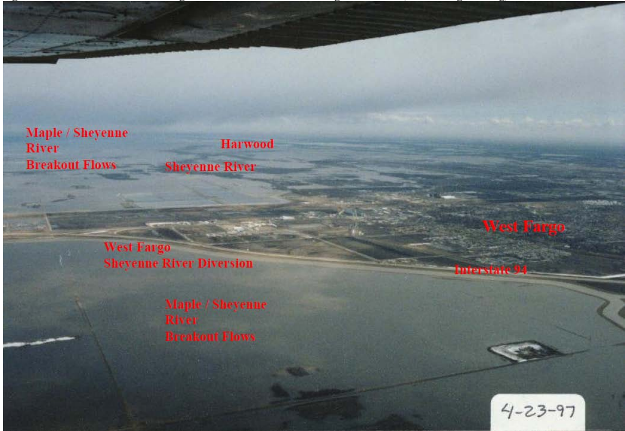
Figure 20. Breakout Flows Looking Northeast near the West Fargo Diversion (Moore Engineering)
