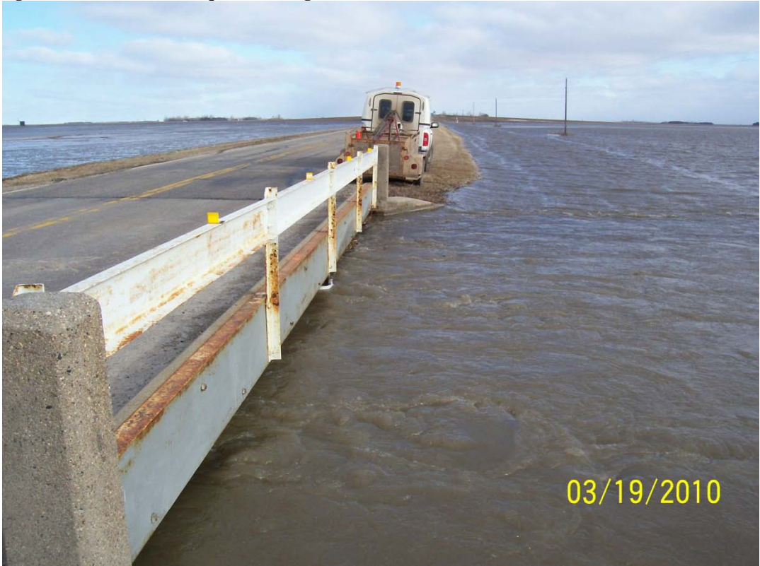
Figure 15. Drain 14 Near Mapleton looking north towards I-94.
