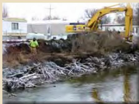
Locally collected red-osier dogwood and willow sod mats were placed on the constructed bench at bankfull elevation.
