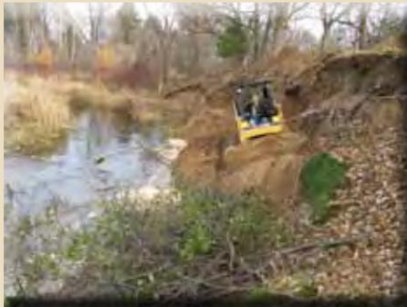
Construction of bankfull bench. A layer of woody debris and fill was placed along the bank toe then covered with live willow cuttings (in foreground).
