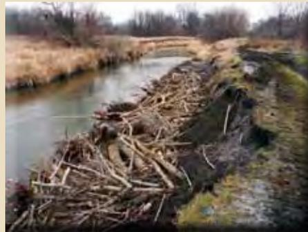
The completed woody debris layer with incorporated root wads. The upper bank was regraded with a more gentle slope.
