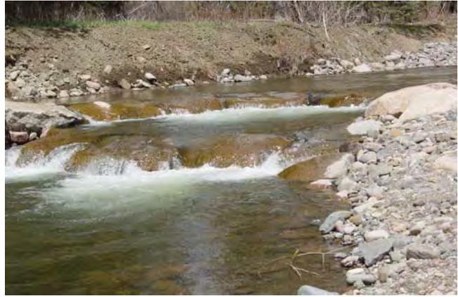
**Figure 11-29** Cross vane structure with step on the East Fork Piedra River, CO
