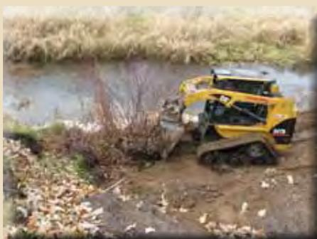
Placement of final layer of sod mats on the constructed bench at bankfull elevation.
