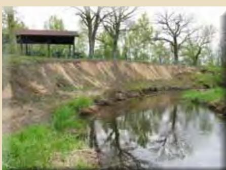
Finished bank stabilization project: Vegetated bankfull bench and a graded streambank protected with erosion control blankets.
