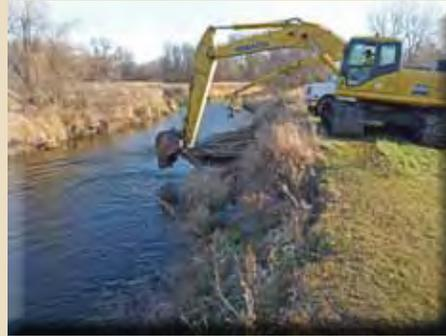
Unstable bank and failing flood control dike protecting a mobile home park. The project started with the placement of woody debris and insertion of root wads.
