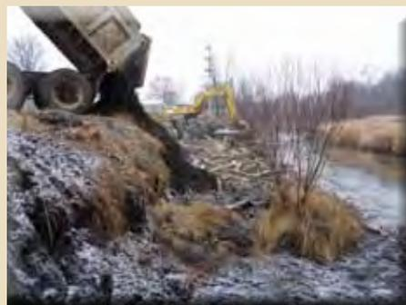
Dirt was added as fill and rooting material to the woody debris layer.
