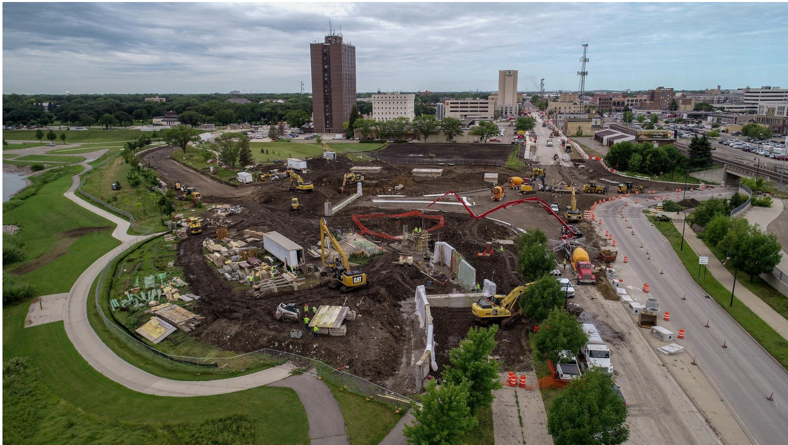
2 nd Street Floodwall – August 14
