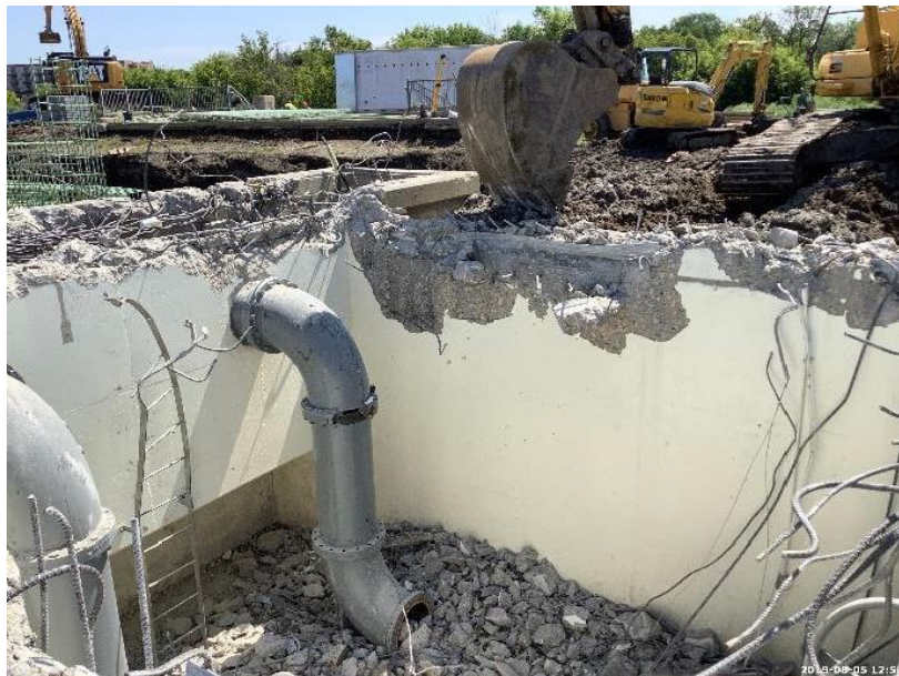
Old Lift Station Removal
