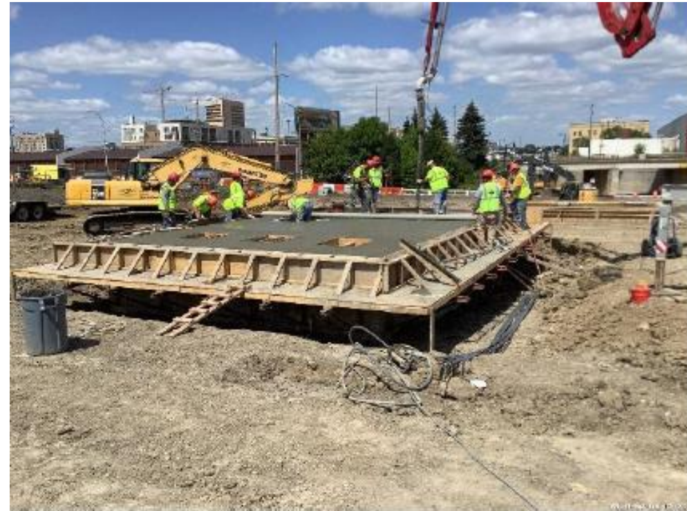
Pump Station Lid Concrete Placement
