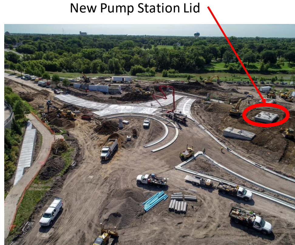
2 nd Street Floodwall – August 21
