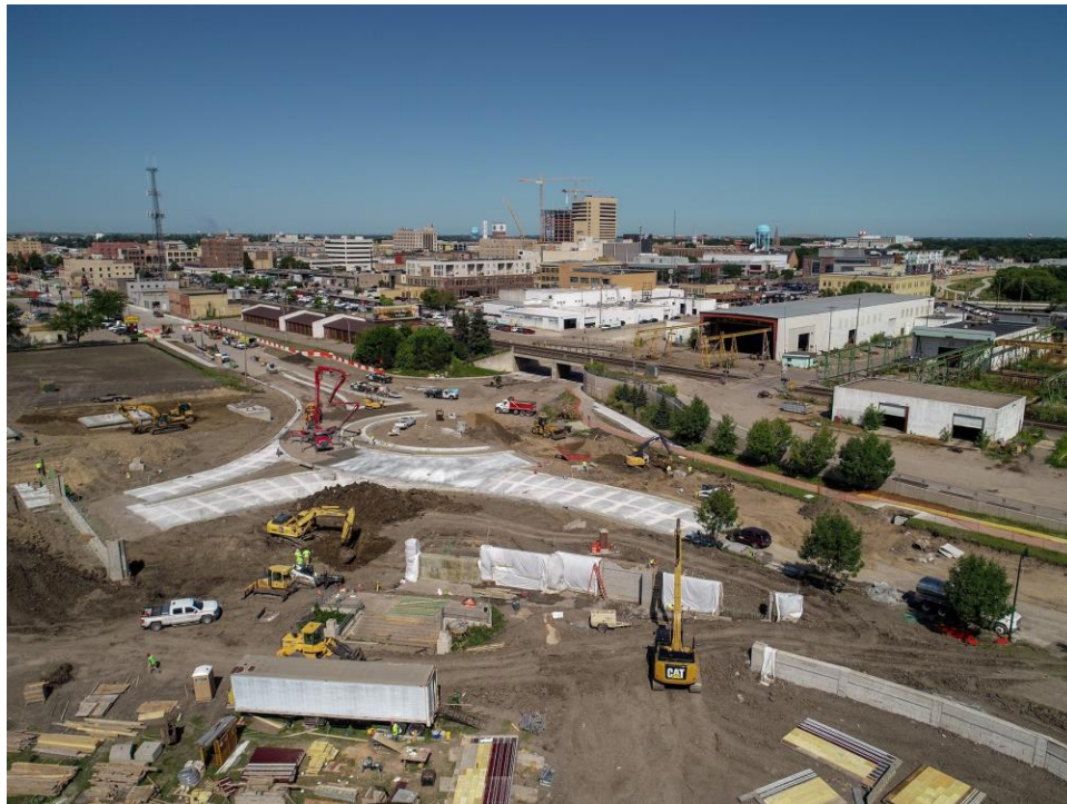
2 nd Street Floodwall – August 21
