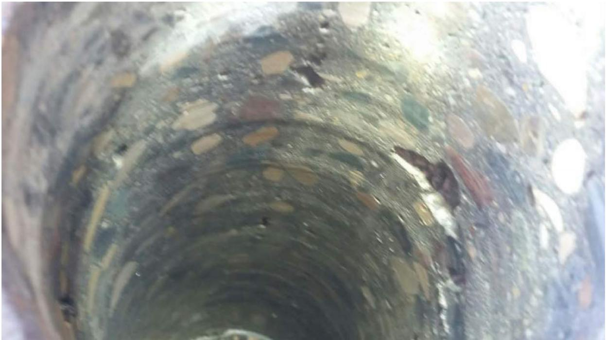
Figure 12: Voids in Core Hole #2
