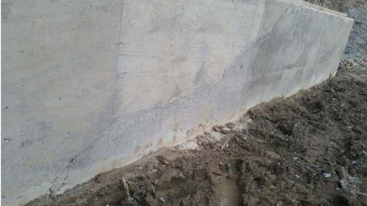
**Figure 3: Possible Cold Joint (looking north)**
