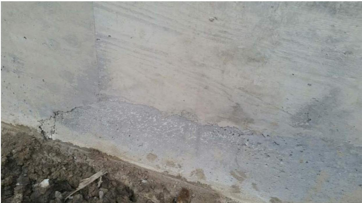
**Figure 4: Possible Cold Joint (near bottom)**
