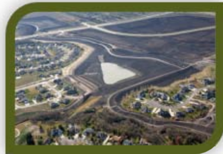
Example permanent mitigation project - Meadow Creek Flood Risk Management Project — 2011
