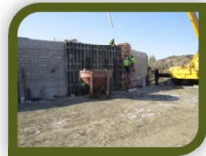
Example permanent mitigation project - Timberline Area Floodwall, Fargo— 2011
