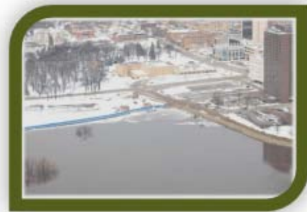
Typical emergency in area of 4 th Street Levee in downtown Fargo — 2009
