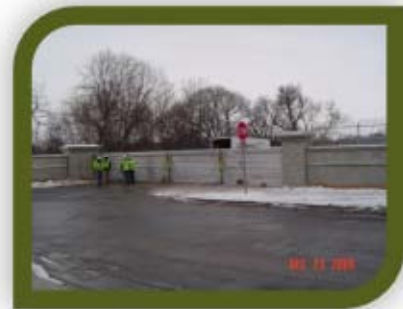
Existing Ridgewood Flood Control Project that would require certification / accreditation
