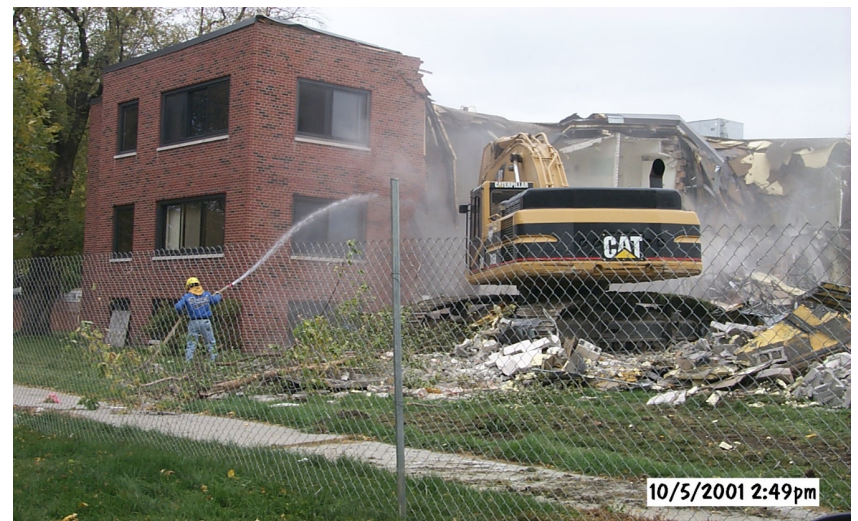
Building Demolition in Grand Forks, ND
