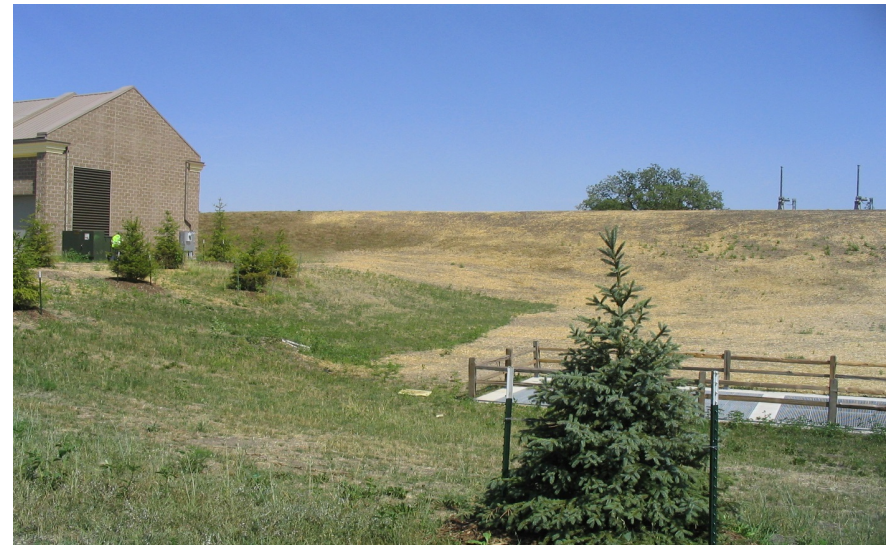
Levee and Pump Station in Grand Forks
