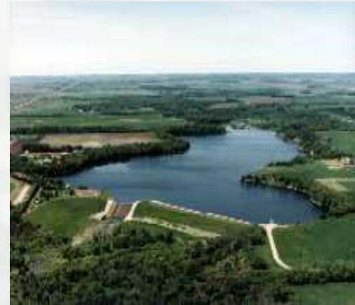
Aerial photo of Homme Dam
