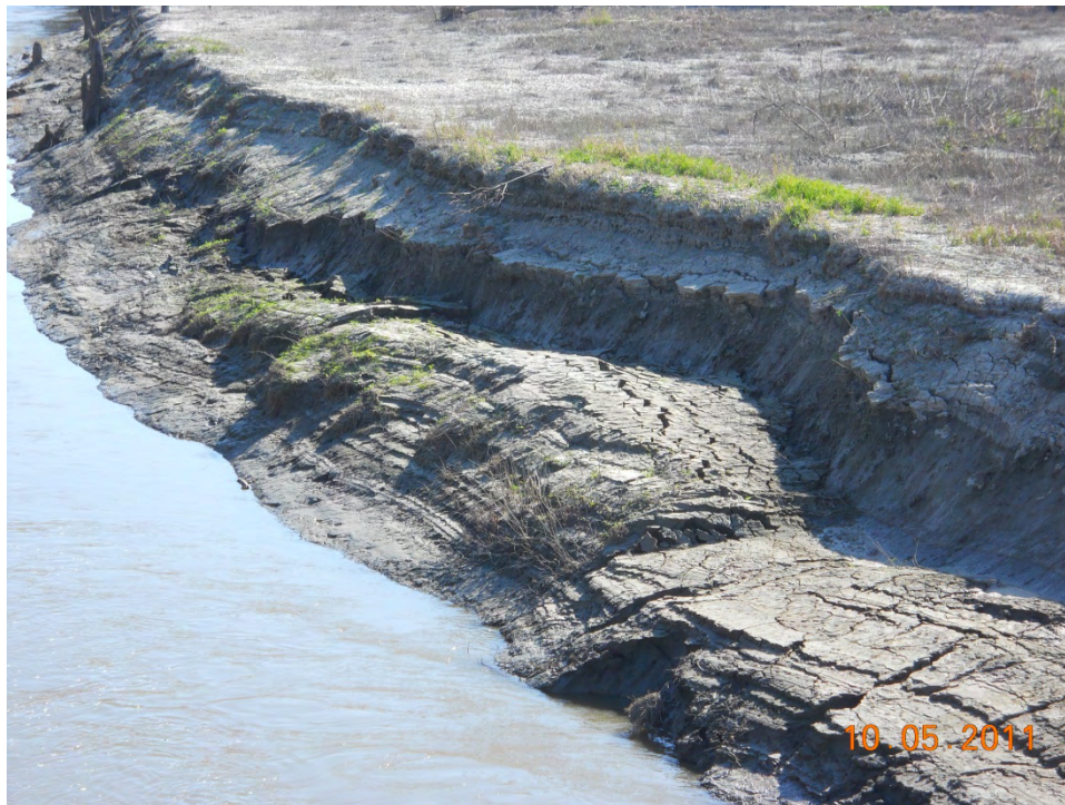
Figure 6-12. Bank Slumping along Sheyenne River - 1
